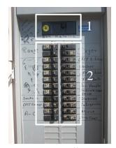
reverse order. While all the branch circuit breakers are off, turn on the main circuit breaker, then flip each branch circuit breaker to the "on" position individually. If you have a backup generator, solar panel array or backup batteries attached to your electrical system, follow the instructions outlined by the manufacturer or installer.
